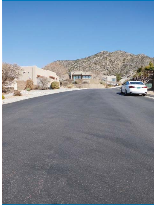
Typical street asphalt
