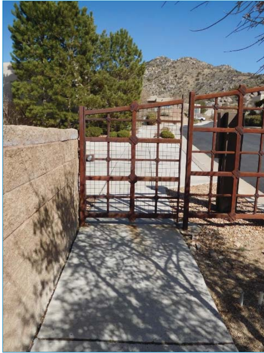
Pedestrian access gate
