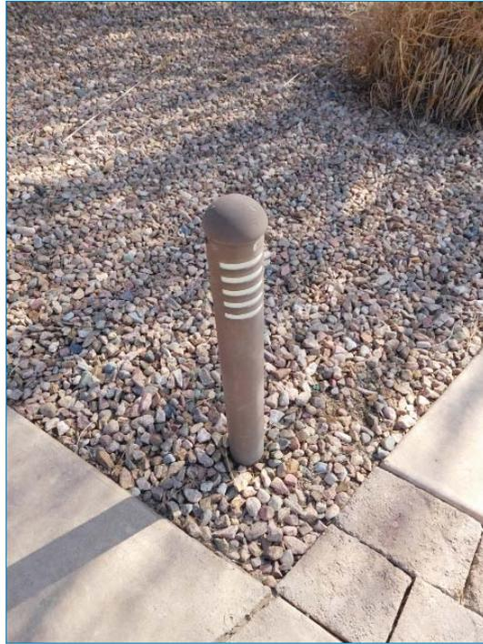
Typical bollard light fixture
