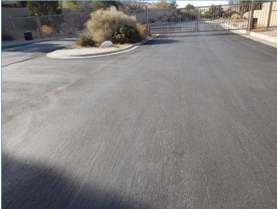
Typical street asphalt
