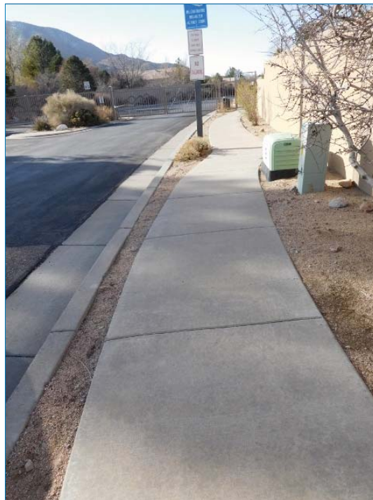
Typical concrete walkway
