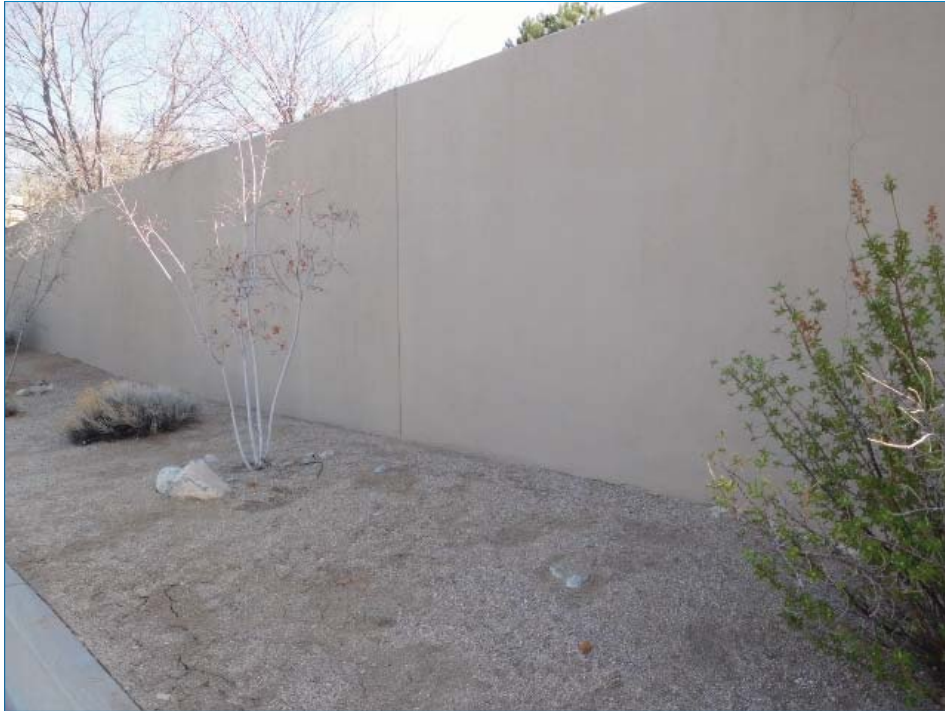
Typical stucco wall
